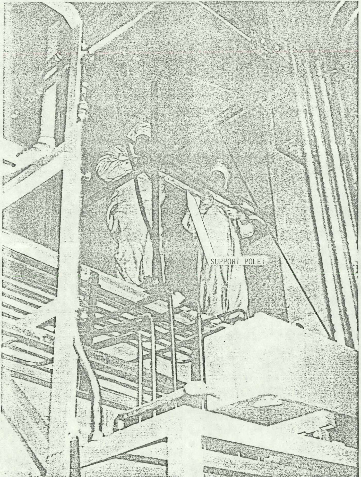
FIGURE 7. Emplacement of SSTR Neutron Dosimeters--Measurement of Reference Point for Stringer Location
